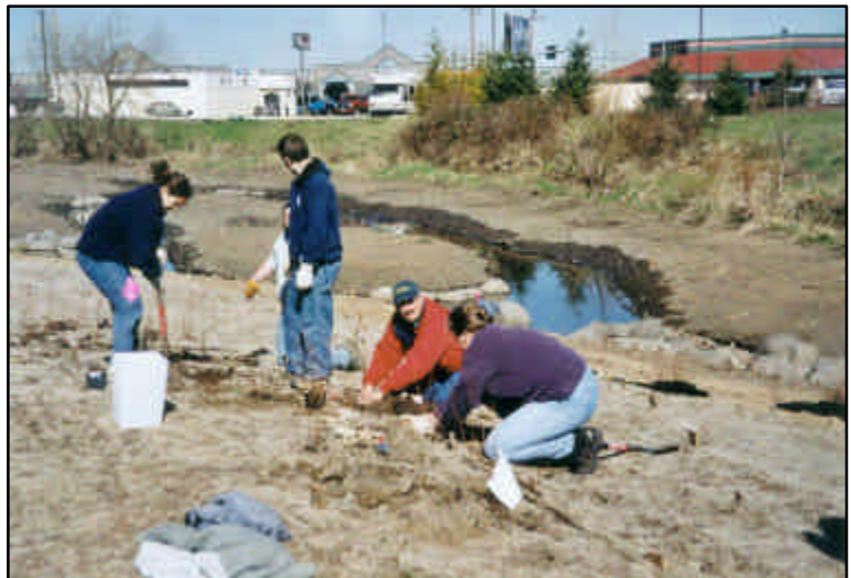
Tree Planting: Feb. 2002- Volunteers from the Council and City of Eugene Stream Team plant hundreds of native wetland shrubs on the newly contoured banks. Jute matting was placed on the exposed soil to reduce erosion while shrubs and grass became established.
