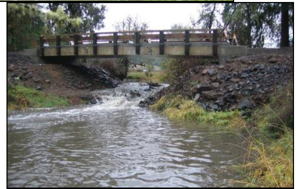
Before & After: The top photo shows the two foot drop at the culvert's outlet in the summer. Now the crossing is passable to fish year round .
