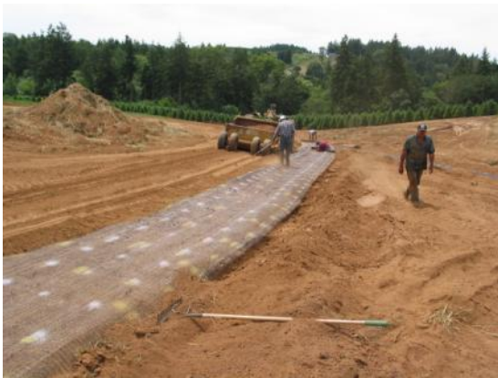
Implementation: The landowner uses a scraper and carry-all to construct the grassed waterway.
