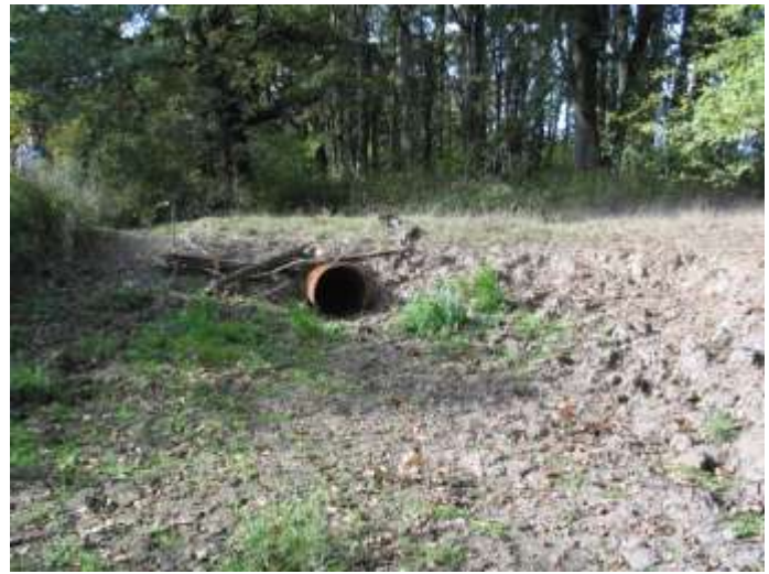
This undersized culvert blocks fish passage on the historic Coyote Creek channel bed.
