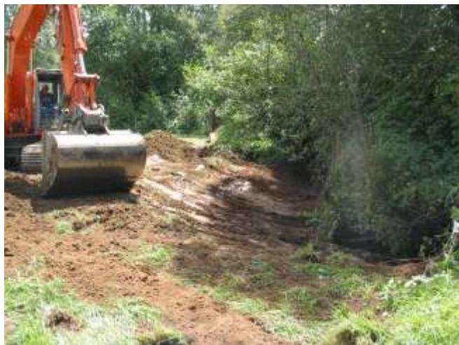
An excavator was used to create terraces at seven sites on
