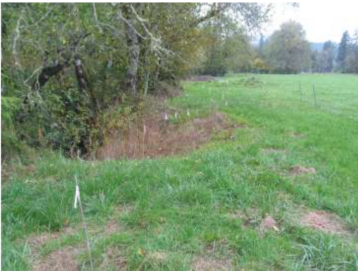
Post-implementation: October 2005- Terrace B has been excavated and planted with native shrubs.
