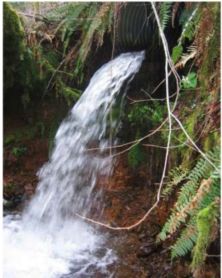
This culvert is significantly "perched", creating a barrier to juvenile and adult fish trying to move upstream.
