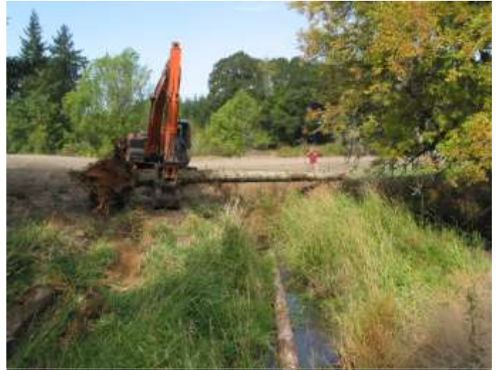
An excavator places logs with rootwads in Owens Creek to provide habitat for cutthroat trout and other native aquatic species.
