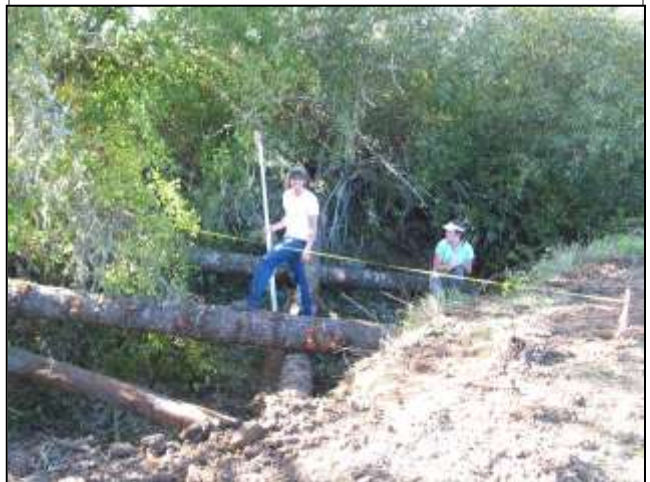
Implementation: Large conifer logs with root wads were positioned in the tributary channel. In addition to enhancing habitat, these logs will help the channel's flow to naturally meander.
