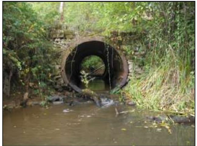
Before the project: Undersized culvert on Owens Creek that will be replaced with a bridge to accommodate crossing vehicle and livestock traffic. **Note that the culvert's outlet is perched above the stream, and its diameter is much smaller than the stream's winter width.**
