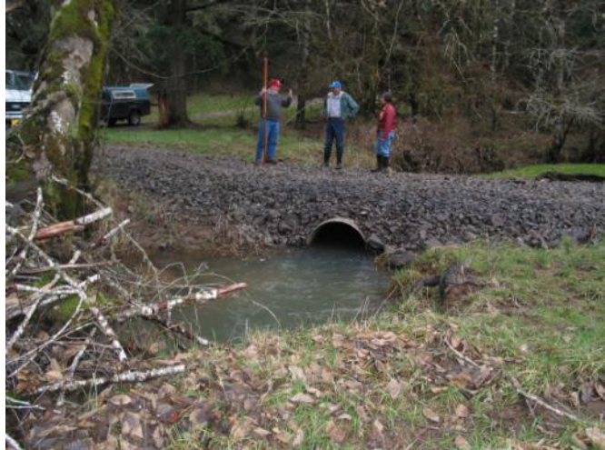
Before the project: This crossing of Eber Creek was a migration barrier for resident and fluvial cutthroat trout and other aquatic species.
