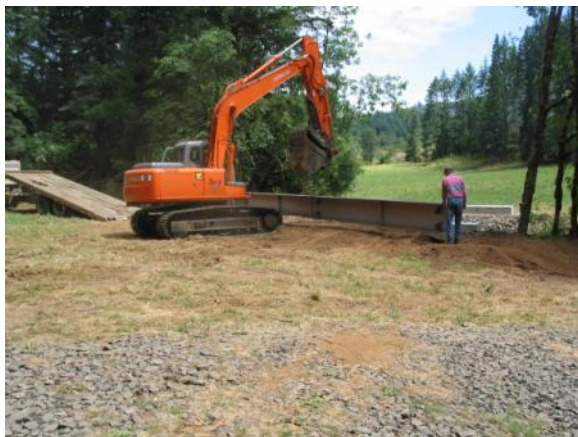
Landowner Andy Thomson assists with the installation of steel bridge supports
