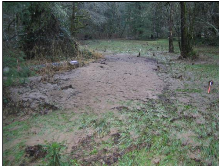
After the project: The large wood has increased overbank flows during flood stage.
