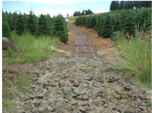
Post-project: view from bottom of drainage looking uphill. This shows the last constructed portion of the grassed waterway, that was completed in June 2010. The bottom of the drainage has a small rock pad that dissipates energy from the sub-surface drain pipe that day lights here.
