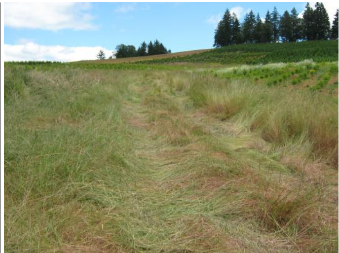
Post-project: Note the much gentler slopes in the drainage area and full vegetative cover. Grass establishment has been excellent.
