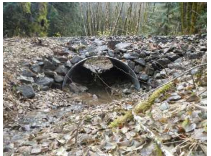
After the project: The barrier culverts were replaced with stream-simulation culverts that allow fish such as cutthroat trout and lamprey, as well as amphibians and mammals, to migrate upstream.
