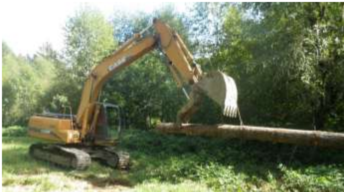
An excavator was used to place logs in Owens Creek.
