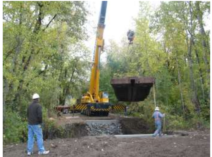
A crane places a railcar bridge over the tributary to Spencer Creek to allow the landowners maintenance access the property on the west side of the tributary.
