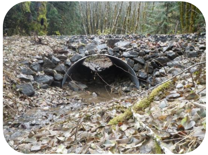
This stream simulation pipe arch culvert opened the upper reaches of Owens Creek for fish passage. Culverts should be as wide as the stream during normal winter flows.
