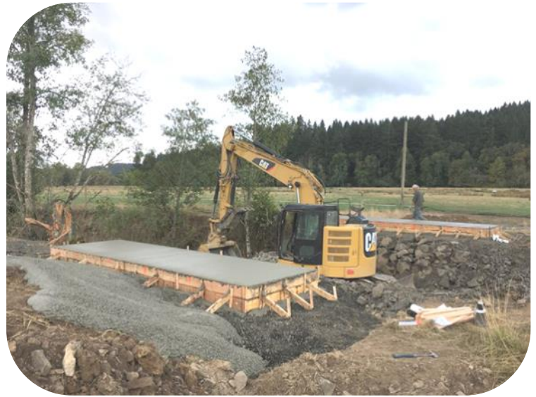
The last priority fish passage barrier on Owens Creek, near its confluence with Bear Creek, was an undersized and perched culvert. Working with Trask Design and Construction, the culvert was replaced with this 40' concrete slab bridge.
