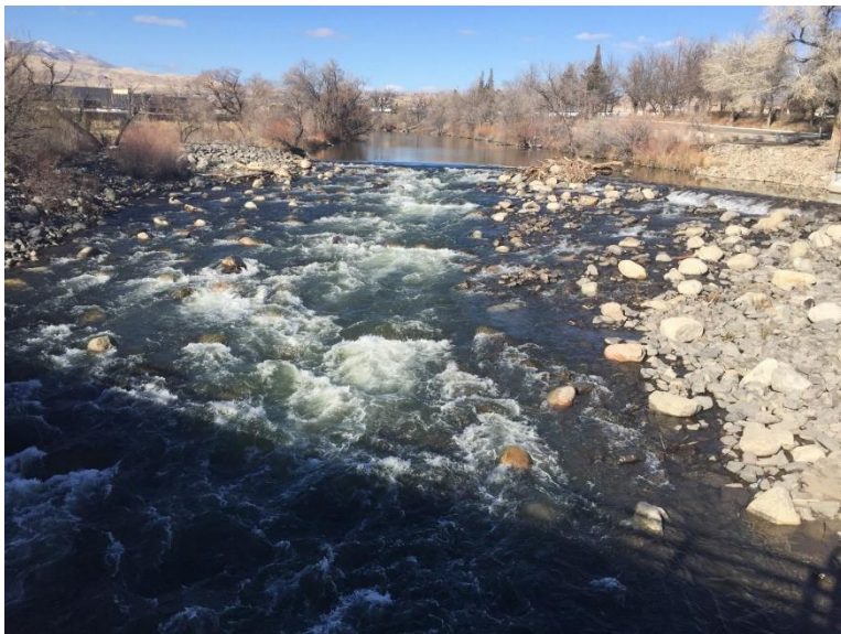
Figure 20. Example of a rock ramp used to modify a low head dam and create fish passage on the Truckee River near Reno, CA.
