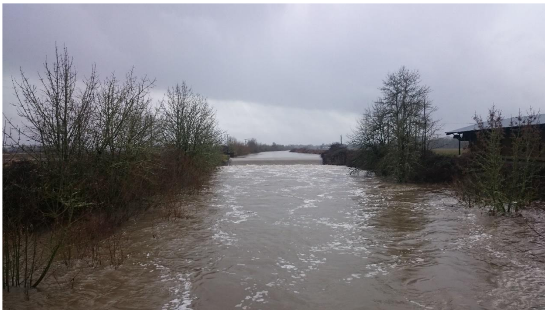
Figure 8. Ferguson Drop Structure – USACE Photo Point 7. Feb 9 2017
