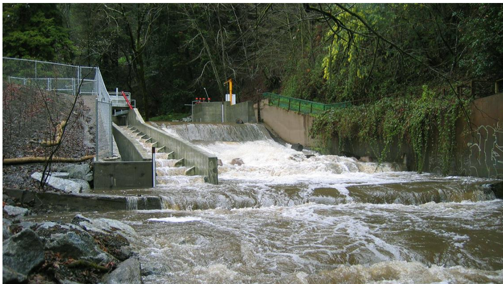
Figure 16. Sample fish ladder built to more recent NOAA standards
