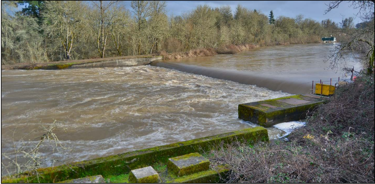
Figure 3-1. The Monroe Drop Structure at high winter flow.
