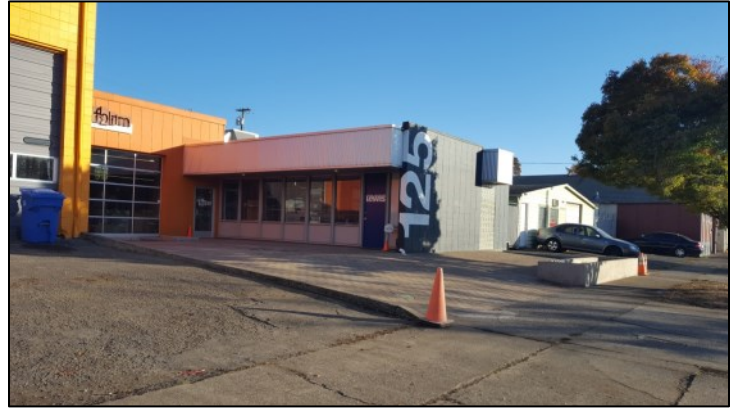
Newly installed permeable paving at 2fORM Architecture
