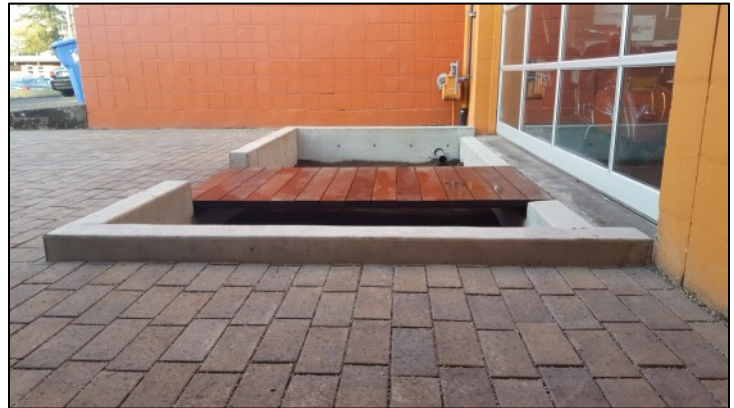
Close up of permeable pavers and bridge over stormwater planter at 2fORM.
