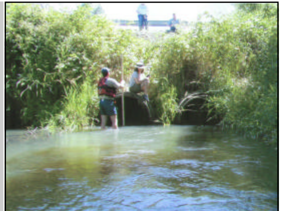
Culverts on Lower Long Tom at Cox Butte
