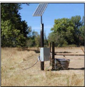
The Bondiolis used a solar powered pump to bring water from Poodle Creek to their off-channel watering station. In the background, you can see the fence they constructed to keep horses away from the creek and riparian area.
