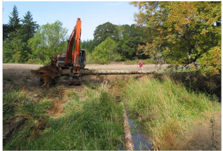
An excavator places logs with rootwads in Owens Creek to provide habitat for cutthroat trout and other native aquatic species.
