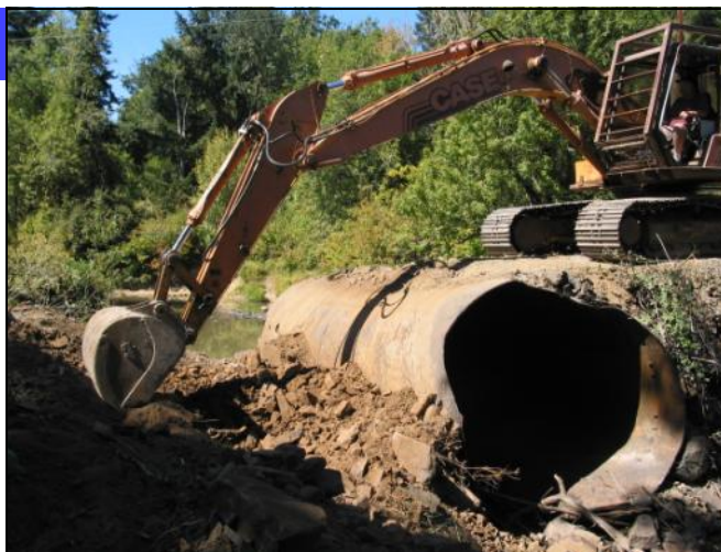
Before: An excavator removes an undersized culvert that blocked fish passage to 46 miles of upstream habitat.
