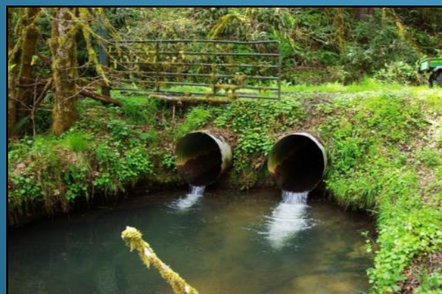
Before the project: The dual culverts of this crossing on Bear Creek were undersized, and their outlets were perched 1.5 feet above the stream.
