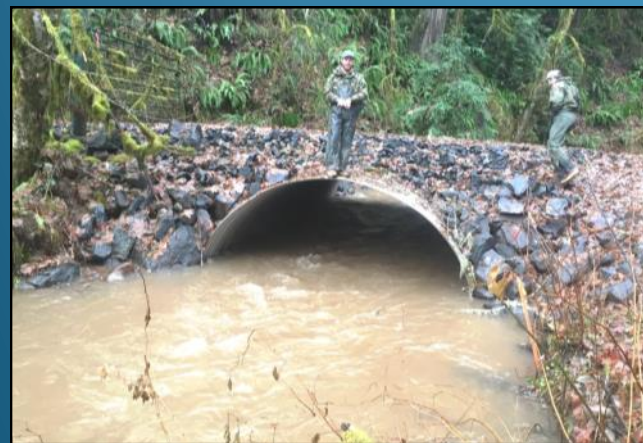
After the project: A single 110” wide culvert can now accommodate winter flows and allow year-round upstream fish passage.
