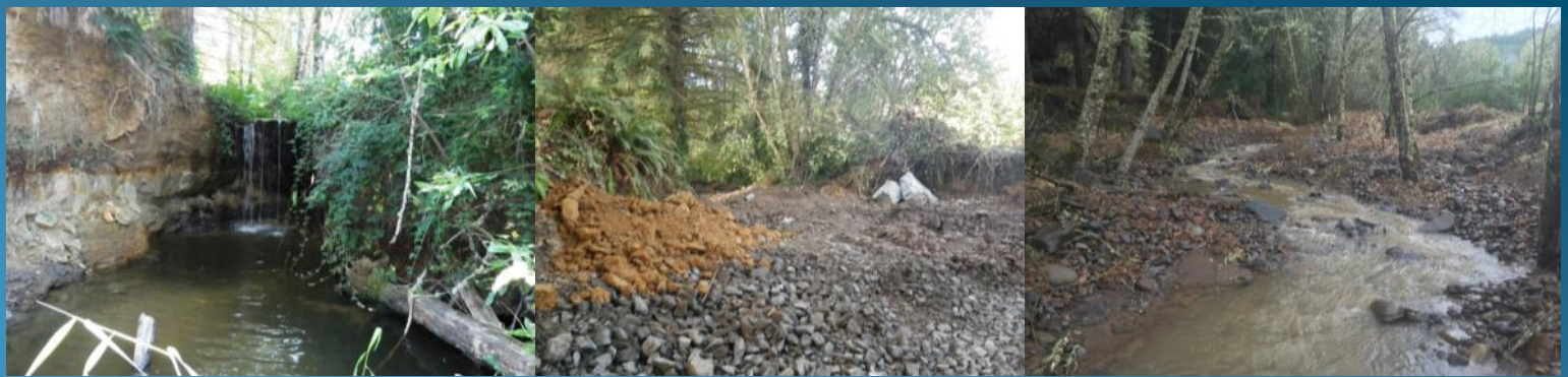
Photos: Vertical 7-foot headcut on Bear Creek blocked upstream access to spawning and cold water refuge habitat (left); Contractors re-graded headcut (middle) into a gradually sloping engineered riffle that allows year-round fish migration (right).
