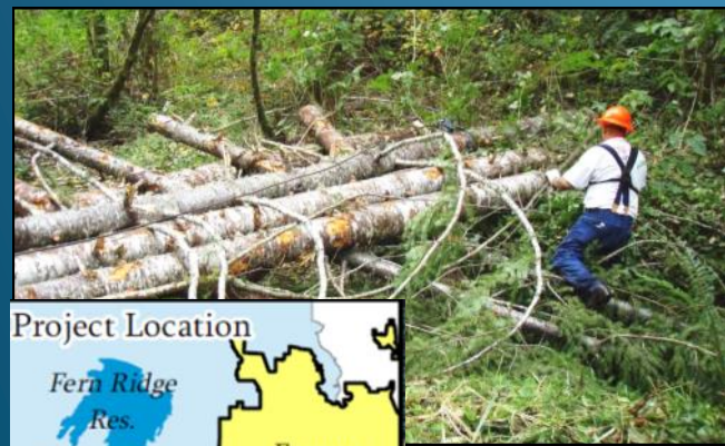
Implementation: Contractor secures cable to conifer in preparation to lift it into stream.
