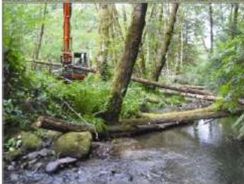
(c) Large wood placement for fish habitat
