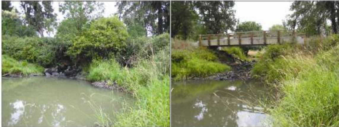
(a) Culvert (before)
