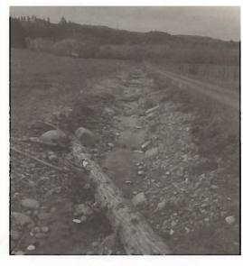
( In this section, the channel was reconstructed with stream rock and log weirs.
