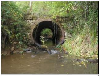
Before the project: Undersized culvert on Owens Creek that will be replaced with a bridge to accommodate crossing vehicle and livestock traffic. Note that the culvert's outlet is perched above the stream, and its diameter is much smaller than the stream's winter width.
