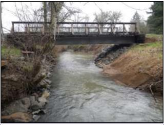
Implementation: This new bridge replaced the undersized culvert at Deck Family Farm.
