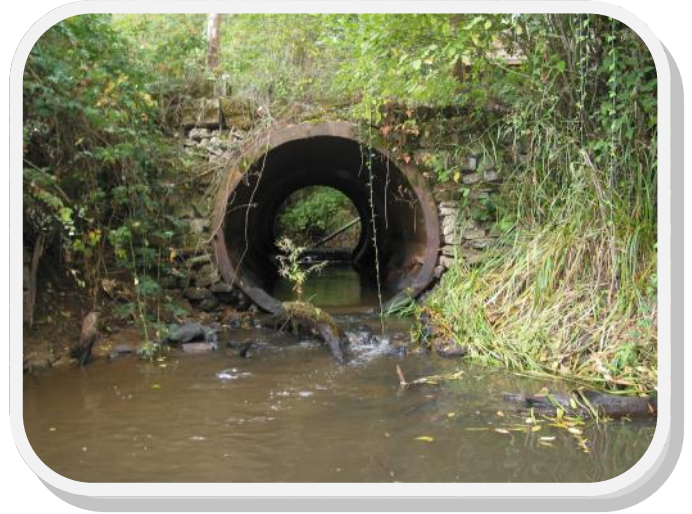
Before the project: Undersized culvert on Owens Creek. Note the culvert's outlet is perched above the stream's surface, and its diameter is much smaller than the width of the stream. ("after" photo on front page)
