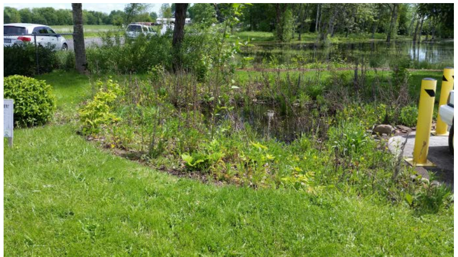
The photo above shows the finished rain garden that sits within a patch of lawn near a storm drain. The lawn and the curb from the parking lot was removed, the drain bypassed, and a depression was created for water to flow into. Native plants have been attracting bees and other pollinators ever since!
