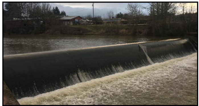
An Army Corps Dam in Monroe Blocks Passage to Native Fish
