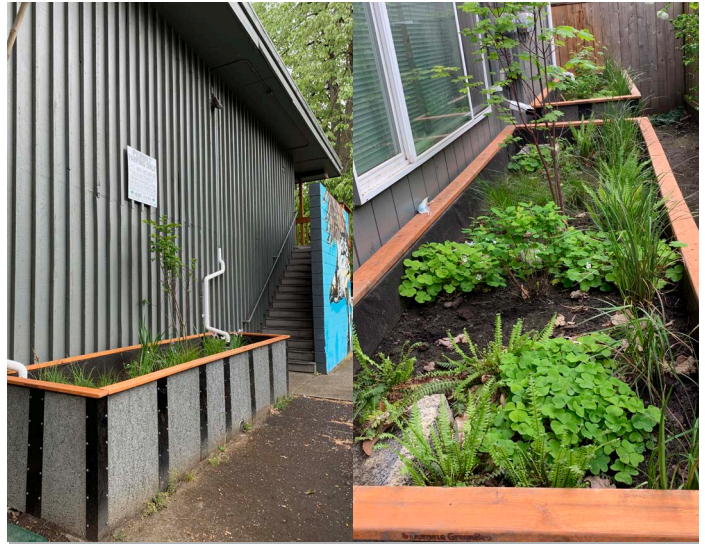
Stormwater Planters at The Monroe, a Veterans Housing unit in downtown Eugene.
