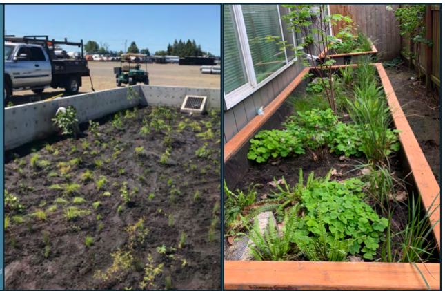
Left: In-ground stormwater planter at Pacific Corrugated (photo: Tim Hahn); Right: planter box at The Monroe
