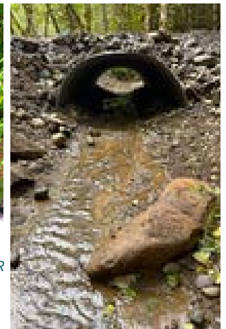
THIS STREAM-SIMULATION CULVERT WAS INSTALLED IN ITS PLACE TO ALLOW YEAR-ROUND PASSAGE FOR ALL NATIVE AQUATIC SPECIES.
