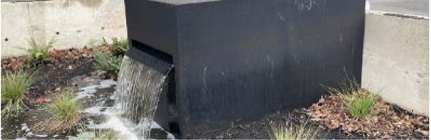
CUSTOM MODIFIED GIBSON STEEL SAND COLLECTOR BASIN, WORKING AS A SEDIMENT DROP FOR THE NEW PLANTER INSTALLATION.
